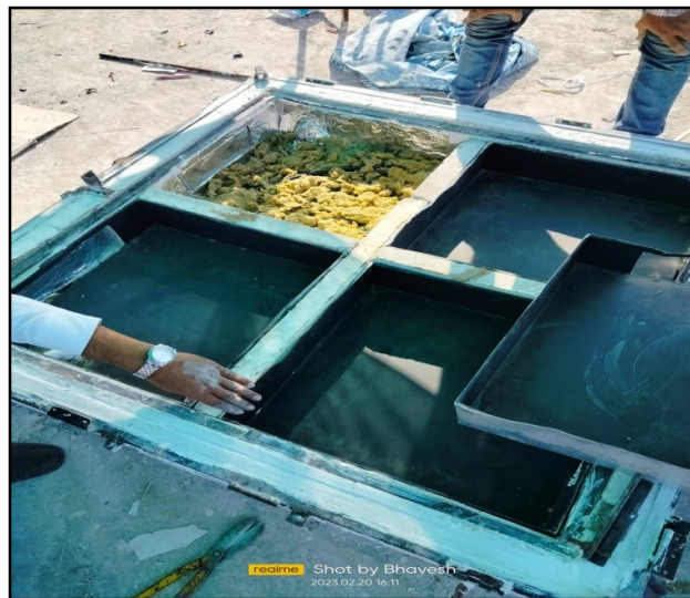
Installation of Chamber
